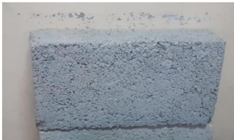
Fig 2: compression failure of concrete block
